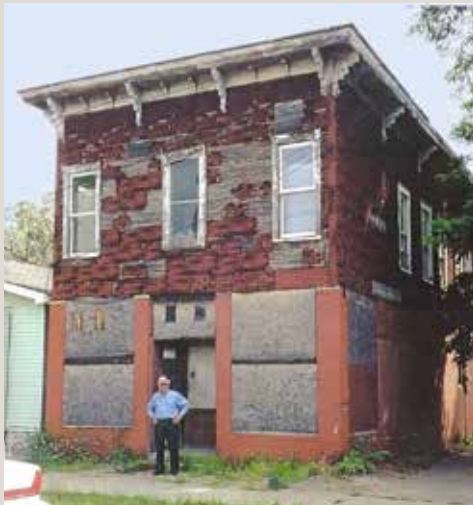
Jamie in front of the building that housed his father's grocery store.
